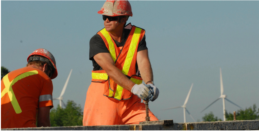
Source: Laborers' International Union of North America (LiUNA!) Renewable Energy
