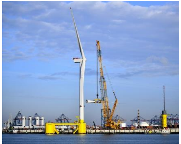
A 9.5 megawatt floating wind turbine for Scotland's Kincardine Offshore Wind project at its assembly dock in the Netherlands in 2021. (Photo: Offshore Wind California / Principle Power)
